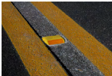
Figure 13 Example of Inlaid (Recessed) Raised Pavement Markers (Source: http://safety.fhwa.dot.gov/roadwaysafetyawards/2013/ )
